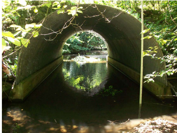
Figure 5: Example of OWEB Culvert Replacement Project
