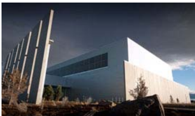
Facebook’s data center in Prineville.
