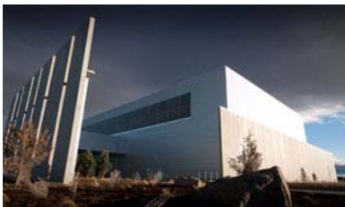
Facebook’s data center in Prineville.
