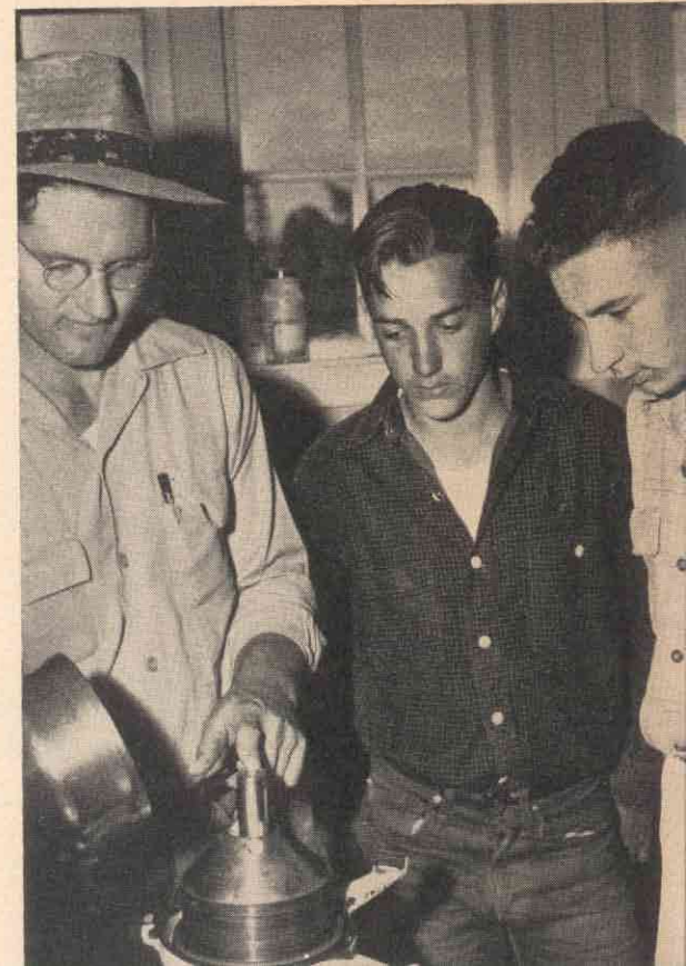
Assembling a Cream Separator
